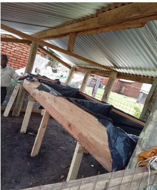
Plate (e). Partitioned vermiculture unit during construction
